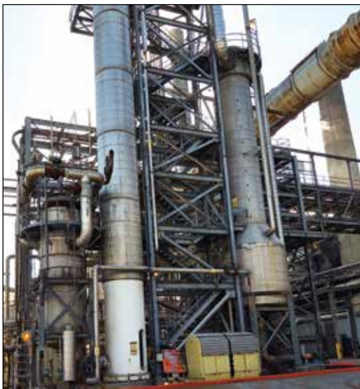
New-Indy Catawba's older steam stripper (left) will remain as a backup to the new system. New-Indy Catawba is the first U.S. pulp mill to have a backup steam stripper.
