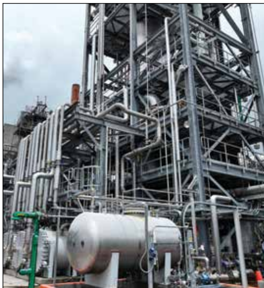
New-Indy Catawba's older steam stripper (left) will remain as a backup to the new system. New-Indy Catawba is the first U.S. pulp mill to have a backup steam stripper.
