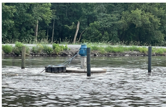
ASB: New-Indy's turbulator helps add oxygen to the wastewater treatment system at the ASB inlet.
