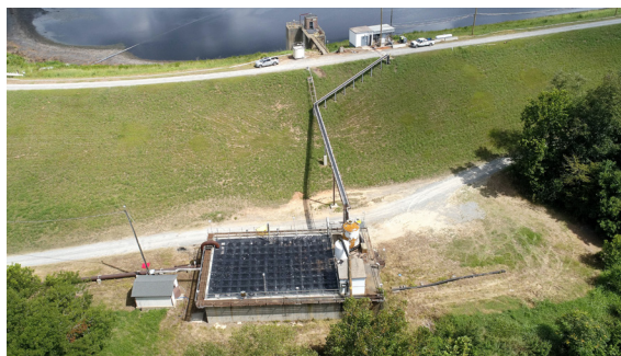
Permanent Cover: A permanent cover was installed on the post aeration basin in June.
