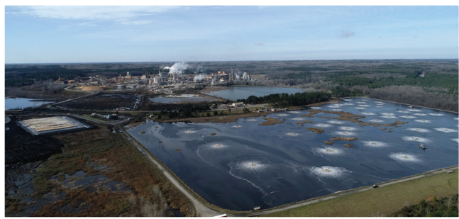
Aeration Stabilization Basin: New-Indy Catawba's Aeration Stabilization Basin operates all 52 aerators 24 hours per day.
