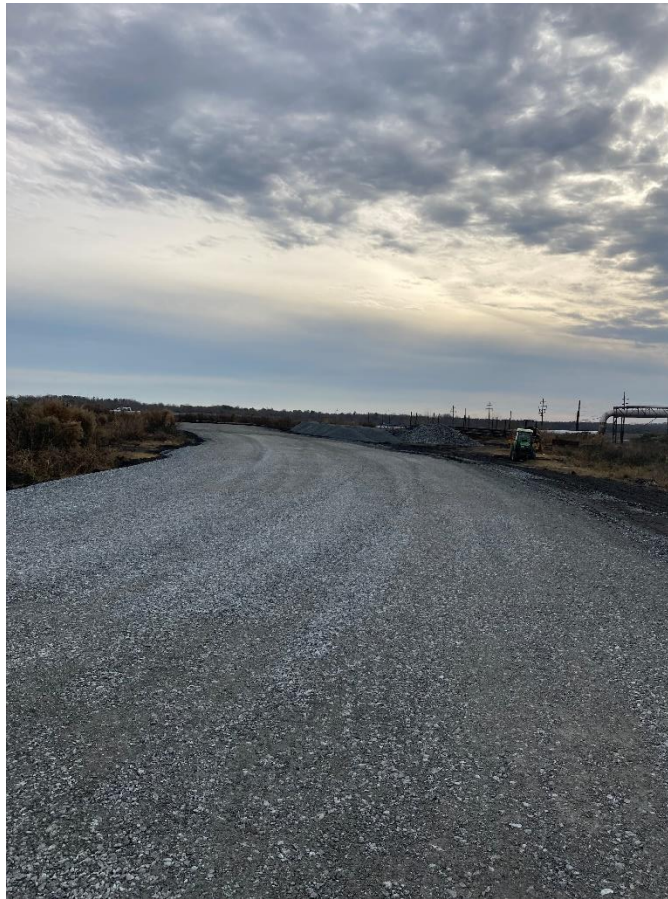
Photo: Haul road improvements to the #4 Sludge Pond.
