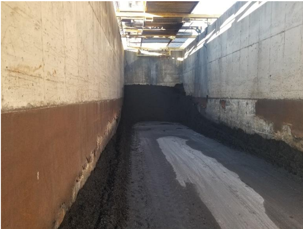
Photo: Ash Storage Bunker.
