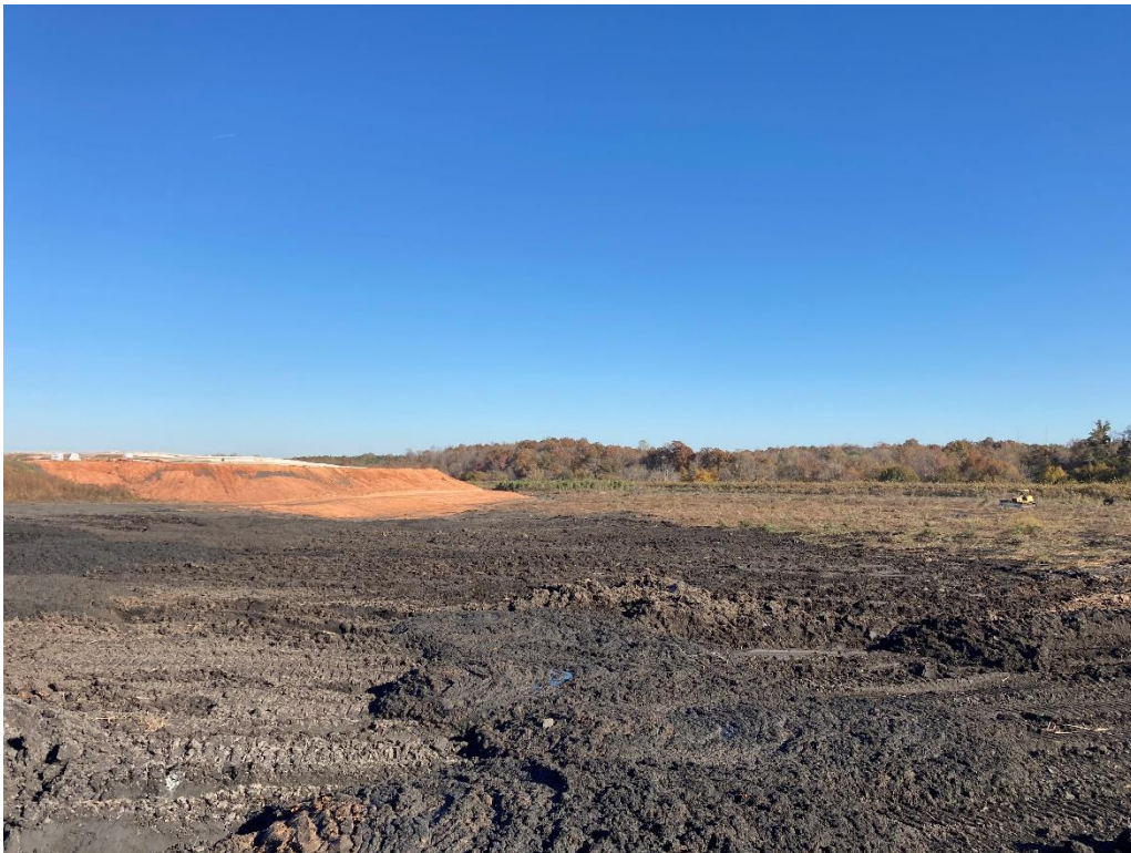
Photo: Sludge Pond #4 cleared to store more waste material.
