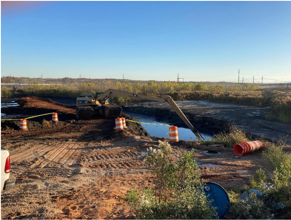
Photo: Floating excavator removing waste material form the EQ Basin.
