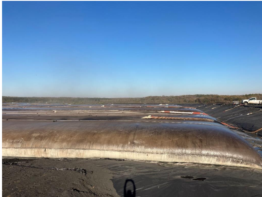
Photo: Geobags used for dewatering solids removed from the ASB.
