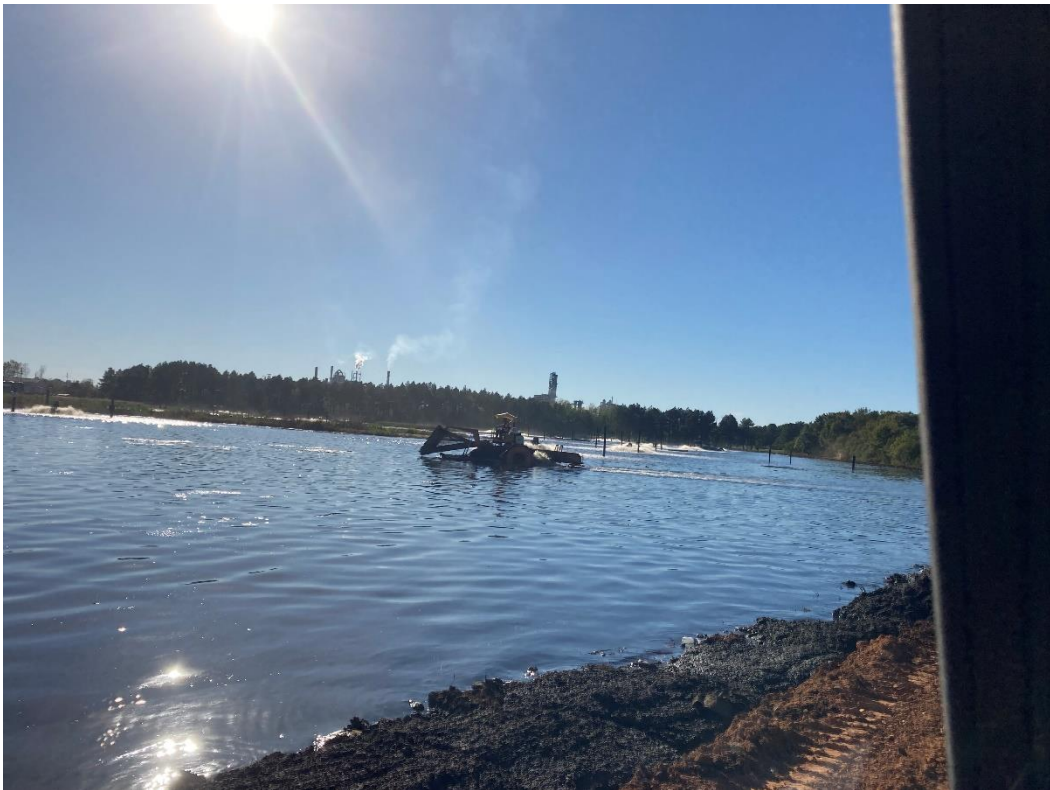
Photo: Weed harvester removing surface material from the ASB.
