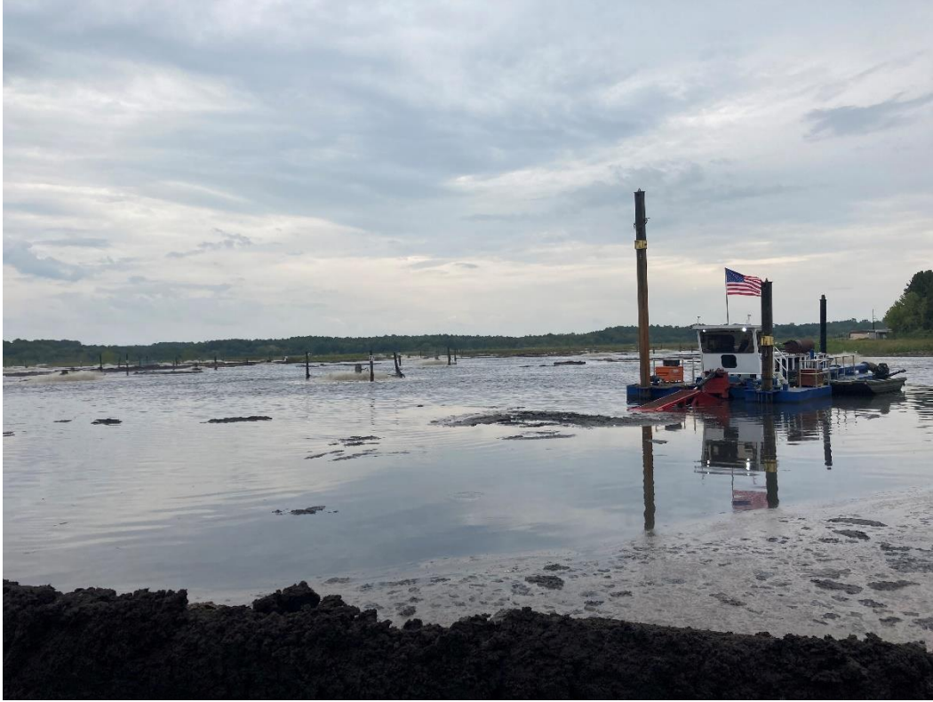
Photo: Subsurface dredge removing solids the ASB.
